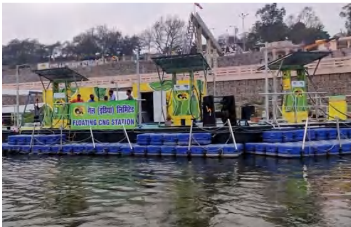
Floating CNG Station for CNG operated Boats, Varanasi
