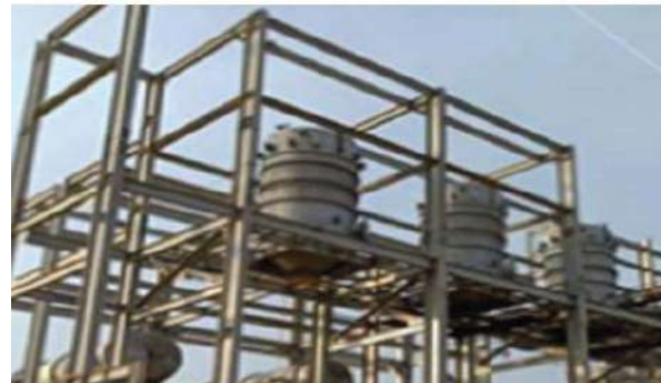
2G Bio-Ethanol Refinery Project at District Bargarh, Odisha
