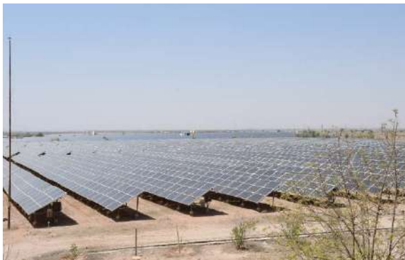
5 MW Rawra Solar Power Project
