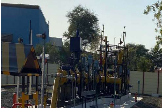
A Typical snap of Hydrogen Blending in the Existing CGD network based on EIL recommendation commenced in Indore City
